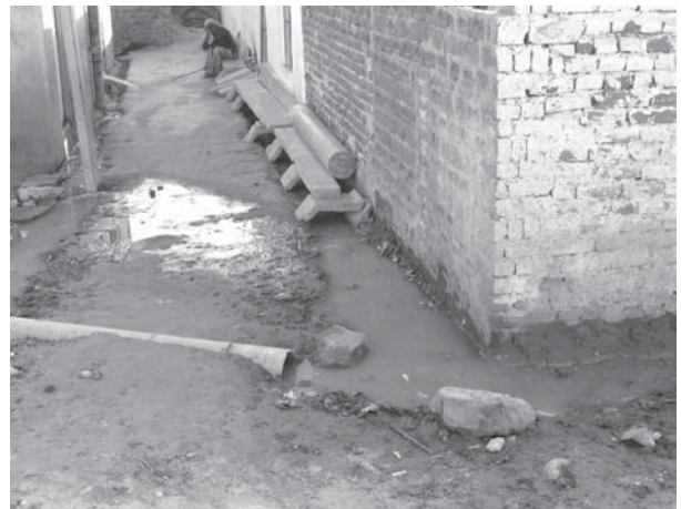
No drains therefore foul smelling sewage water flows through the streets in Kacchi Basti
